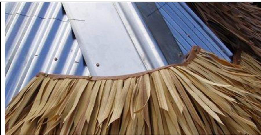
An **additional** Fiber Bali tile (400mm) is fitted **half way** between the guide lines on the roof to ensure that an even thickness is maintained on all hip corners.
