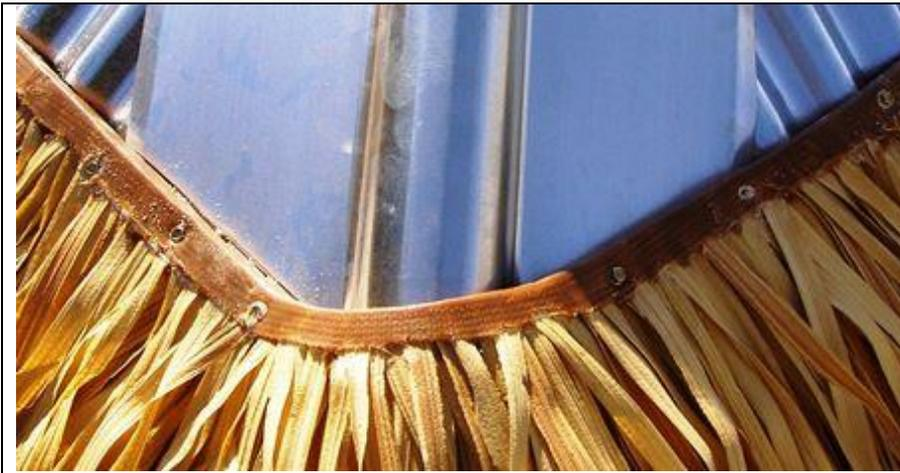
The flexible polyurethane backing of the Fiber Bali tiles is easily bent over the hip caps to create a tight appearance.
