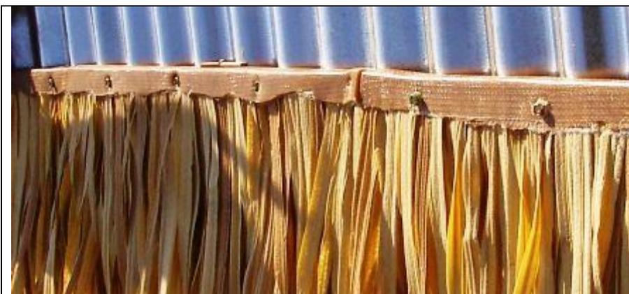
Fasten the screws **until the screw head is flush** with the polyurethane backing strip of the tile. Six screws / staples required per tile, spaced at 160mm.
